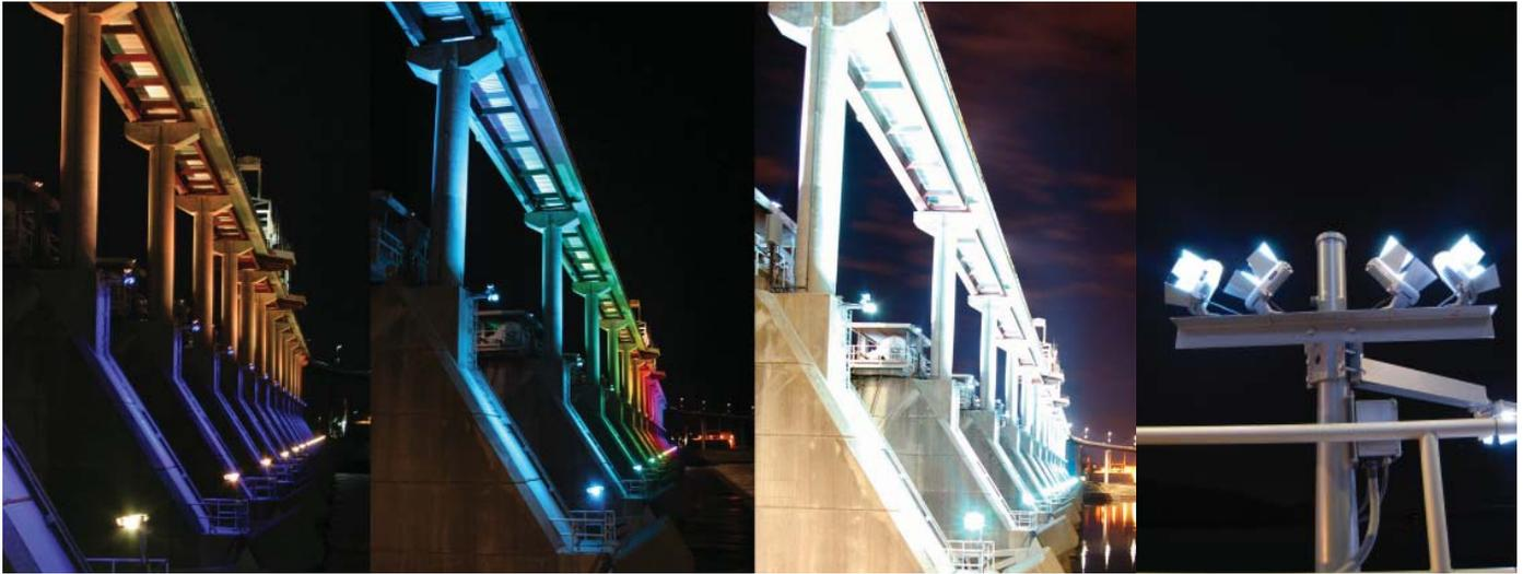
Second, the LUXEON LEDs give the lamps a life expectancy of at least 50,000 hours compared to only 10,000 to 15,000 hours for a metal halide solution. Given the number of fixtures and the challenges of changing them in the Big Dam Bridge's outdoor environment, this dramatically reduces both replacement costs and maintenance requirements.
